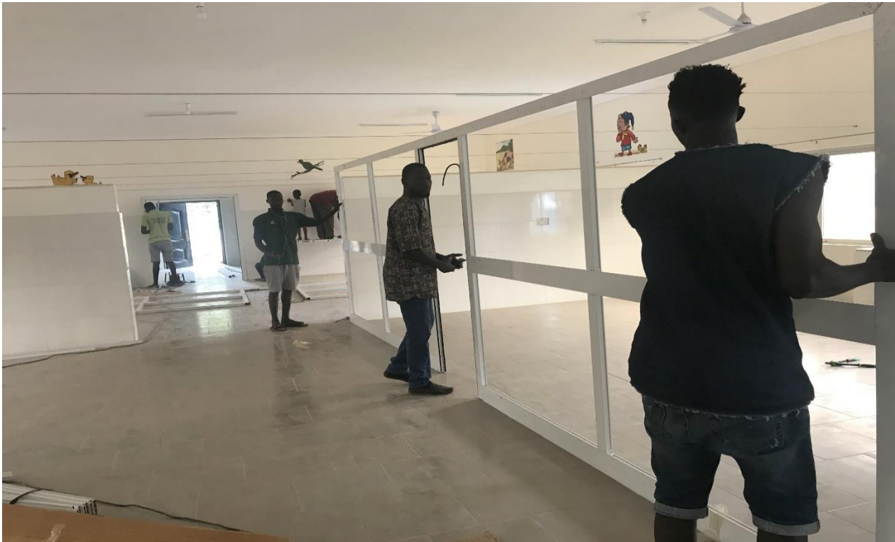
Installing ward partitions in the renovated children's unit
